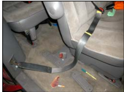
Figure 11. View of second row right safety belt anchor
