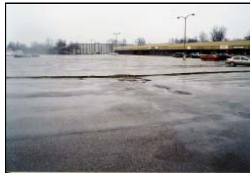
Figure 2. View of parking lot and concrete sidewalk
