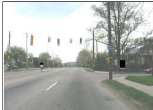
Figure 4. Oldsmobile approach to intersection.
