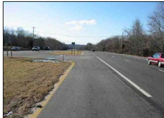
Figure 2 - Westbound approach of Mazda 626.
