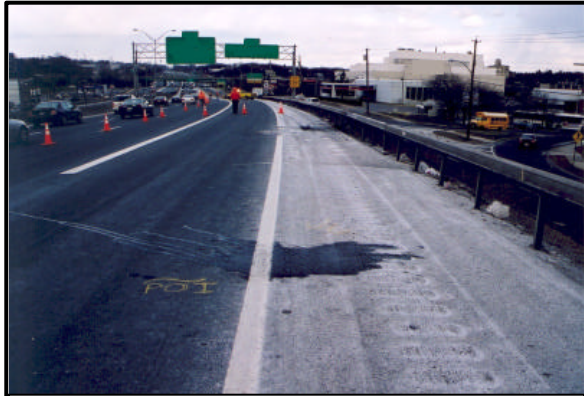
Figure 4: Point of impact.
