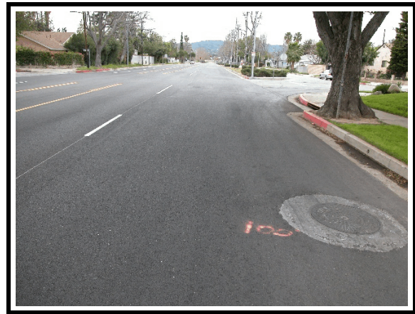
Figure 2. Approach to area of impact (south)
