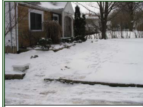
Figure 4. Struck retaining wall and sidewalk steps.
