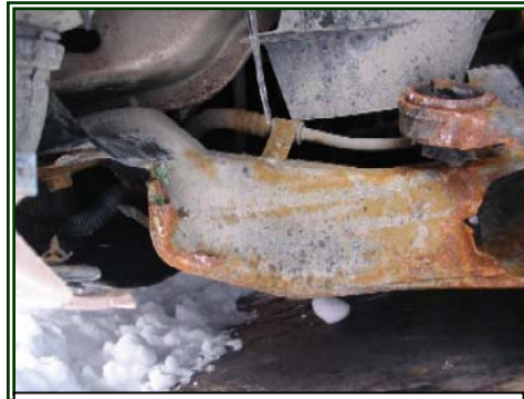
Figure 8. Crushed leading edge of the left frame rail and separation of the lower control arm.
