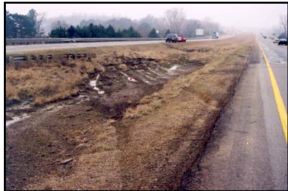
Figure 3: Westward trajectory view of the Ford into the center median.
