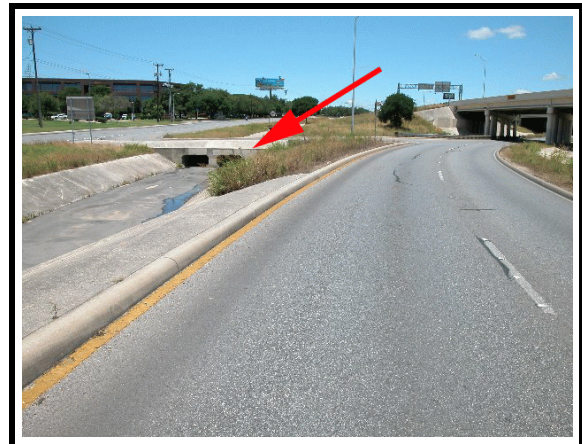
Figure 1. Area of road departure. Impact is marked with red arrow.
