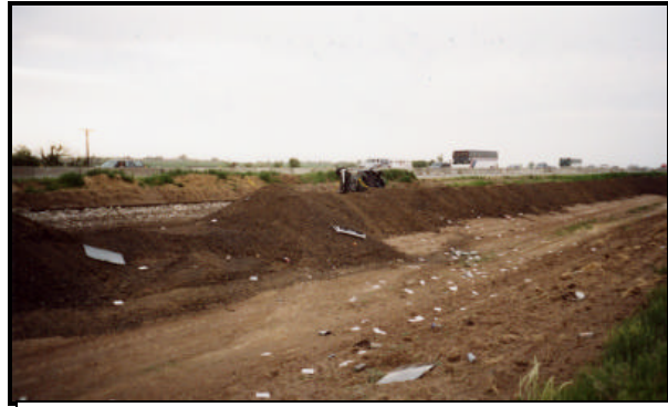
Figure 3: Northwest view across the median from the edge of the northbound lanes.
