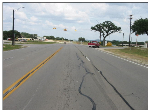
Figure 2: Hyundai's east-northeasterly path of travel in inside northeastern lane approaching four-leg intersection (case photo #05)
