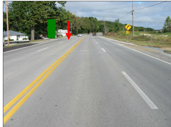
Figure 1: Case vehicle's north-northwestward travel path in inside northern lane; Note: arrow shows approximate point of impact (case photo #02)
