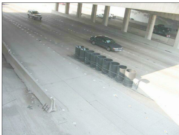
Figure 4: Impact area–Nissan hit barrels (1 st event), case vehicle impacted Nissan (2 nd event), and case vehicle’s left rear impacted barrels (3 rd event); Note: barrel type and/or configuration likely different from date of crash (case photo #07)
