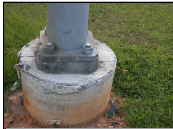
Figure 5: View of the concrete base support.
