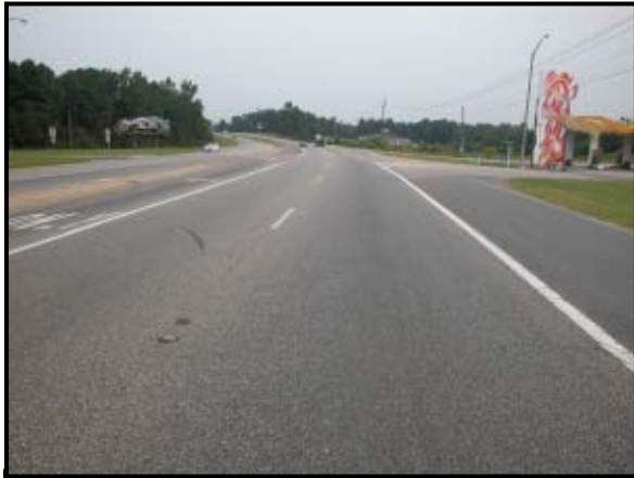
Figure 2: Eastbound view approaching the intersection.
