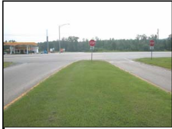
Figure 3: Southbound view of the intersection.
