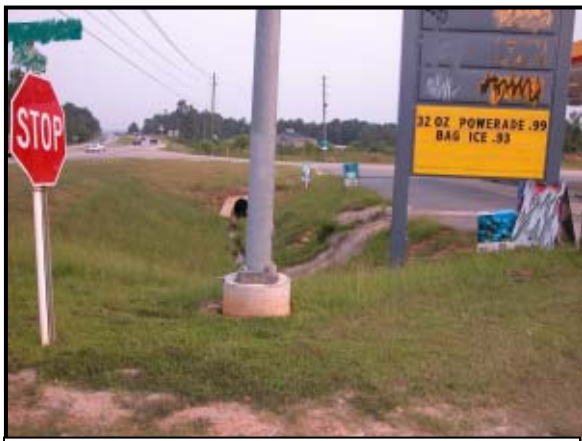
Figure 4: View of the SE intersection quadrant and the area of final rest.
