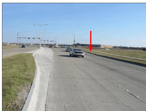
Figure 1: Case vehicle's east-southeasterly travel path in inside through lane of eastern roadway, approaching four-leg intersection; Note: left-hand curvature, beginning of left-hand turn lane, and beginning (arrow) of right-hand turn lane (case photo #01)
