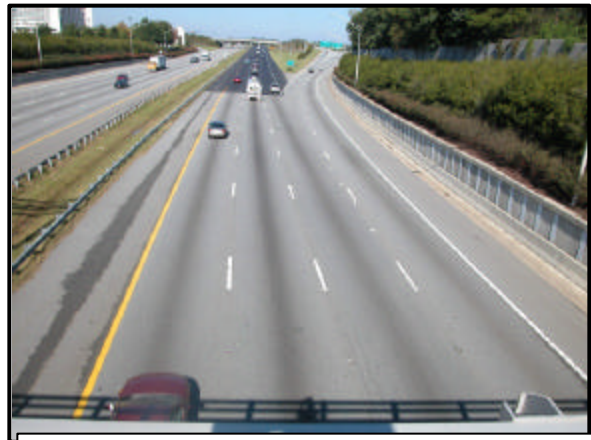
Figure 3: Westbound view of the repaving project.
