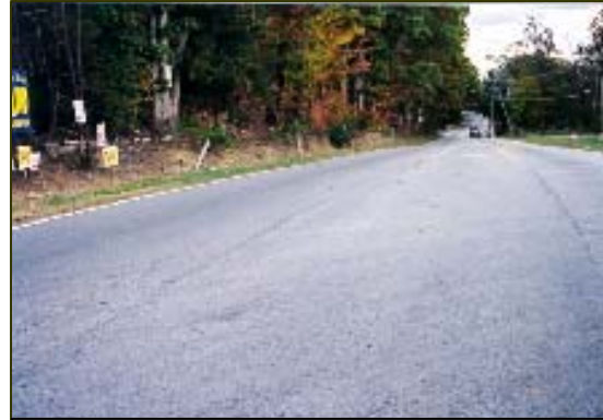
Figure 2. Overall southbound view of the crash site.
