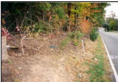
Figure 4. Impacts with the embankment and numerous small diameter trees.
