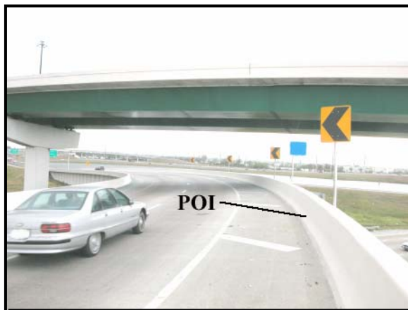
Figure 2: Southwesterly view at the point of impact.
