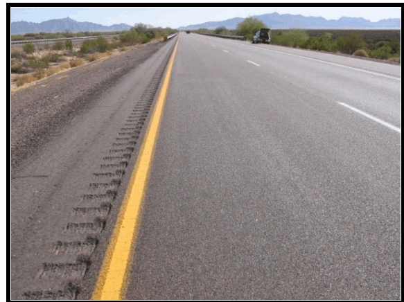
Figure 1. Approach to impact with guardrail end treatment—east
