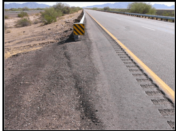
Figure 2. Impact with end treatment (replaced)
