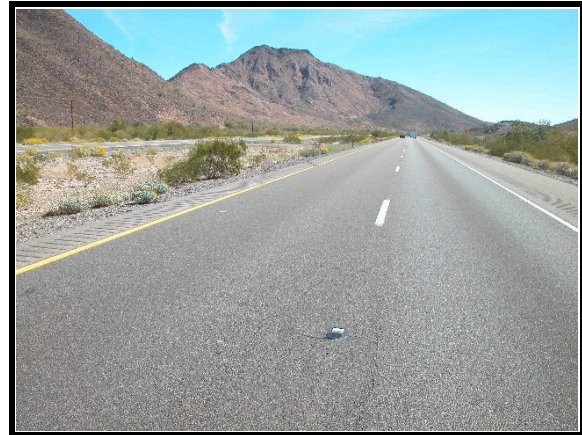
Figure 1. Approach to left hand road departure
