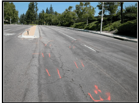
Figure 4. Area of rotation and vehicle overturning - case vehicle
