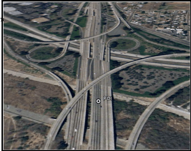
Figure 3. Overview of roadway—looking toward the north
