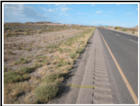
Figure 3. Area of road departure-left side (eastbound)
