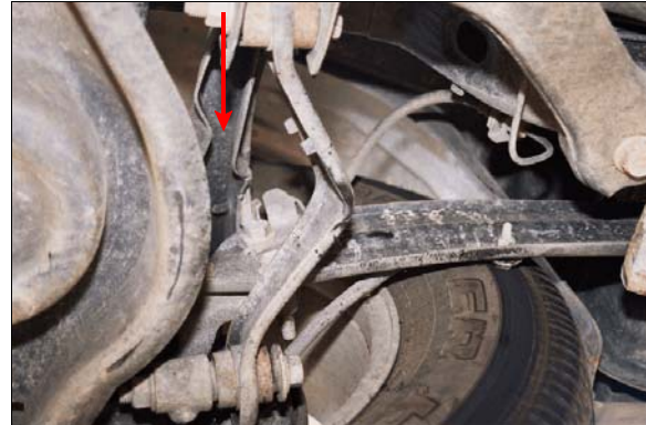
Figure 20: Left rear wheel contacting trailing arm, toe link bent in V-shape, arrow points to bent upper control arm
