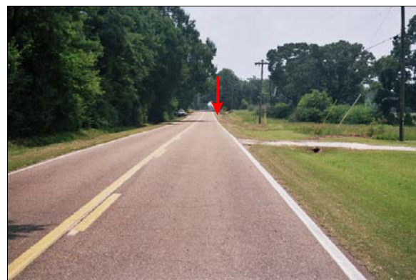
Figure 1: Approach of case vehicle in southeast bound lane, arrow shows area of rollover
