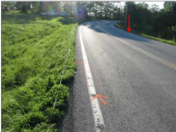
Figure 4: View west to left rear yaw mark on south edge line of roadway (orange arrow), red arrow shows area of second right rear yaw mark
