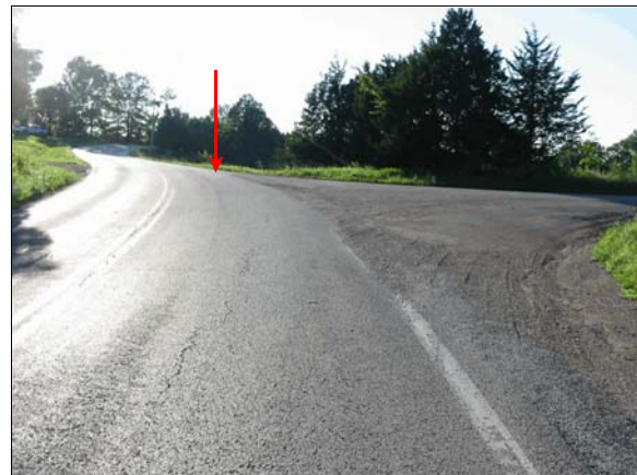
Figure 2: Intersecting roadway with loose gravel, arrow shows area of first right rear yaw mark
