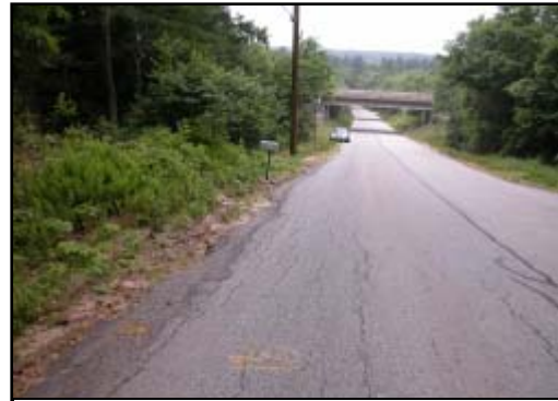
Figure 2. Westbound view of crash site.
