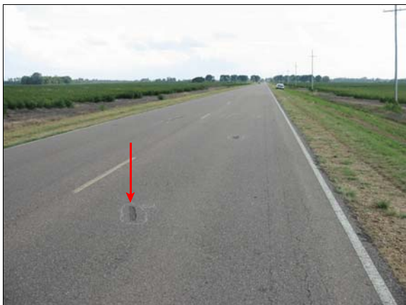
Figure 3: Angled gouge indicated by arrow shows area of impact in southwest travel lane
