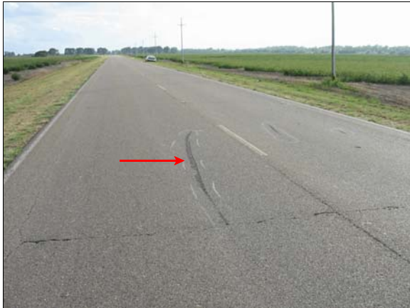
Figure 5: Arrow shows pavement gouge from rim of case vehicle's left front wheel
