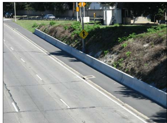
Figure 3: View to northeast to area of case vehicle's sideswipe impact with the concrete longitudinal barrier (case photo #02)
