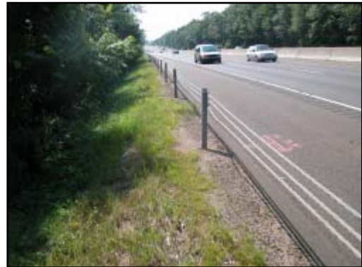
Figure 2. Close-up of three-strand cable guardrail (northbound roadside)
