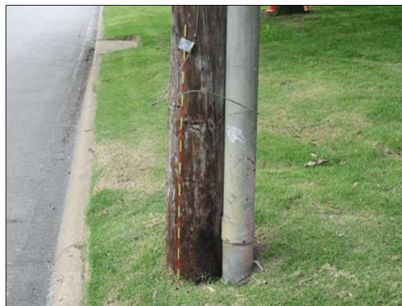
Figure 5: The utility pole [each stripe on rod is 5 cm (2 in)], case vehicle impacted steel conduit pipe (case photo #04)
