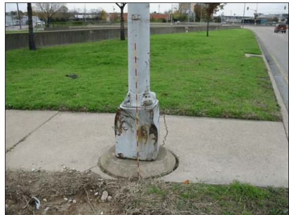
Figure 6: Traffic signal pole impacted by case vehicle, dent in base of pole is old damage
