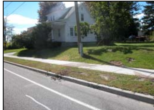
Figure 5. West roadside curb impact.
