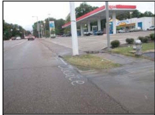
Figure 2. View of crash site and concrete light pole
