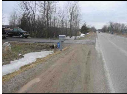
Figure 3 - Area of road departure.
