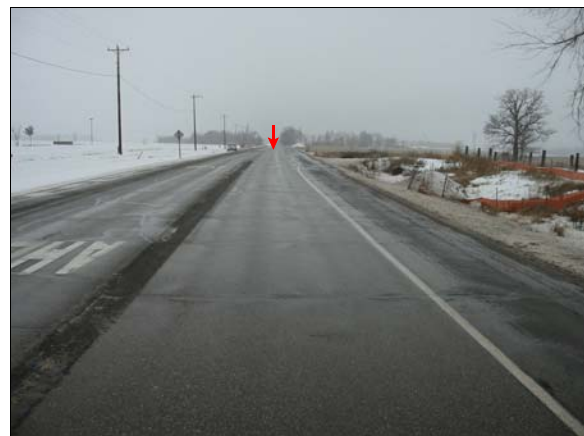
Figure 1: Overview of the trafficway and approach of the school bus southbound to impact, arrow shows area of impact
