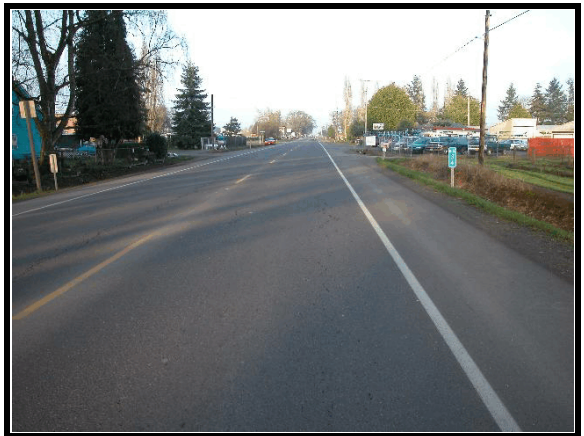
Figure 2. Approach to area of impact - north
