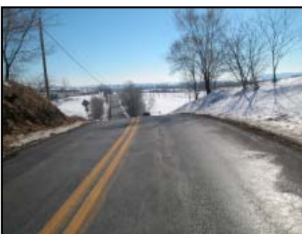
Figure 3. Southbound approach at hillcrest and left curve
