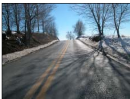
Figure 2. Southbound approach to the hillcrest and left curve
