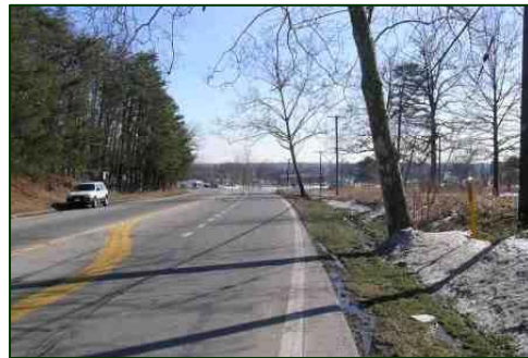
Figure 2. Southbound approach to the crash site.
