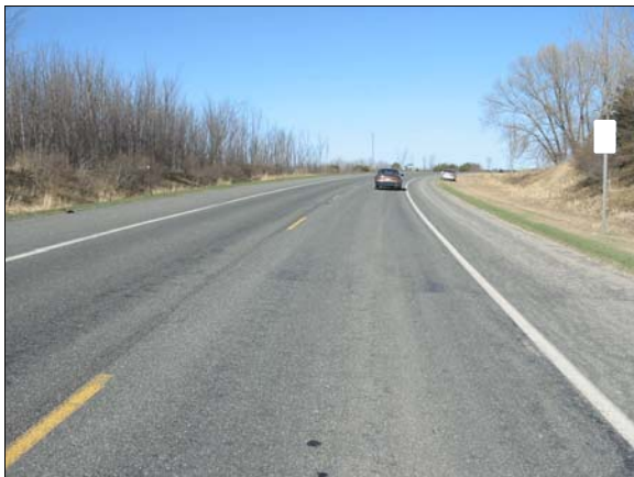
Figure 1: Overview of case vehicle's northeastbound approach
