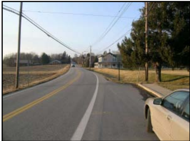
Figure 2: Northbound trajectory view at the crash site.
