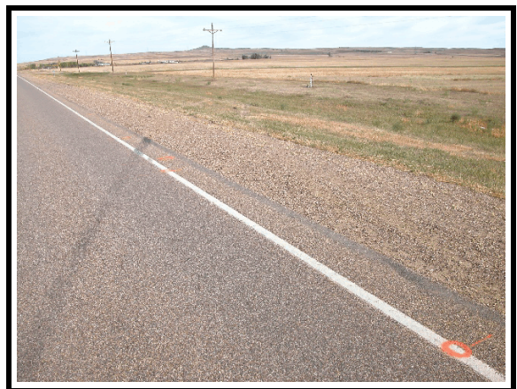
Figure 3. Area of roadway departure
