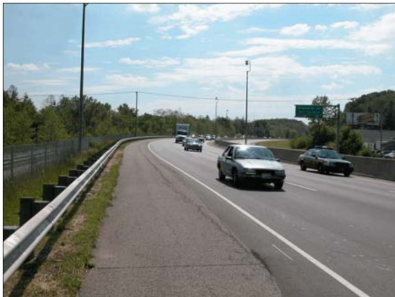
Figure 1: View to southwest at case vehicle's approach on the divided highway, photo taken adjacent to mouth of exit ramp
