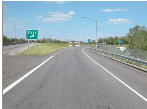
Figure 2: Approach of case vehicle northeastbound on the exit ramp
