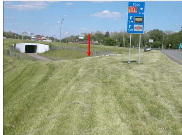
Figure 4: Approach of case vehicle to impact (arrow) with back, top section of bicycle tunnel header wall
