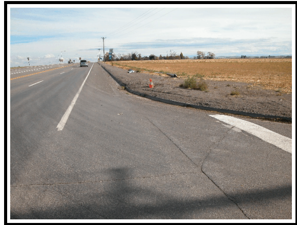
Figure 3. Path to impact with light pole
