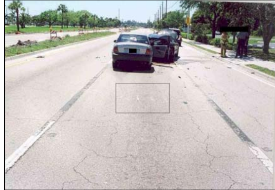
Figure 3 - Area of impact with gouging on the asphalt roadway.
