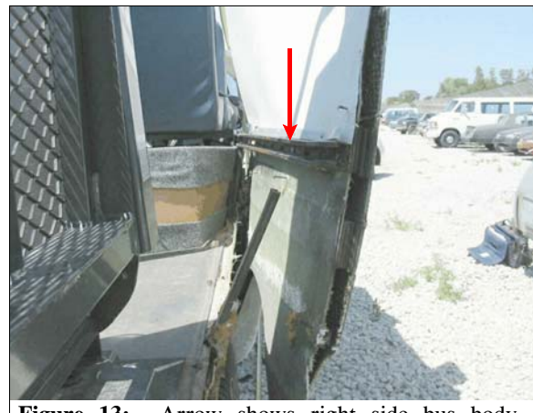
Figure 13: Arrow shows right side bus body screwed to metal frame that runs length of passenger compartment.
