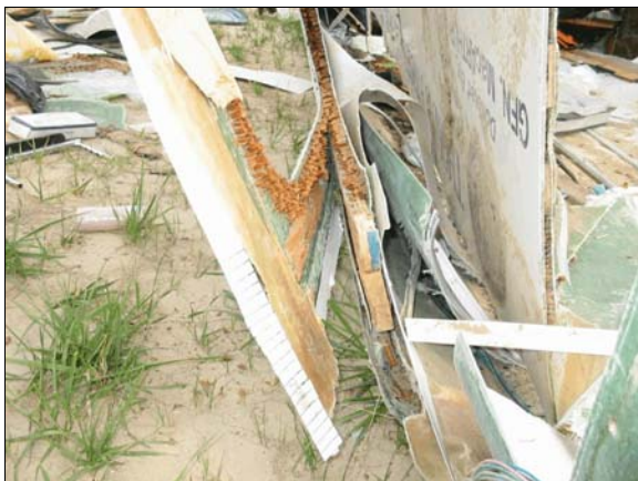
Figure 12: View of left front of bus body showing wooden frame and fiberglass construction
