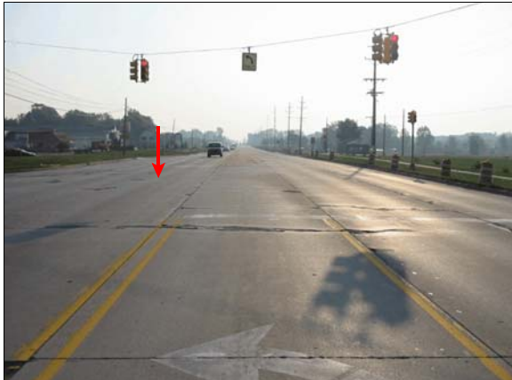
Figure 2: Approach of the Chrysler Sebring eastbound in the left turn lane, arrow shows area of impact
