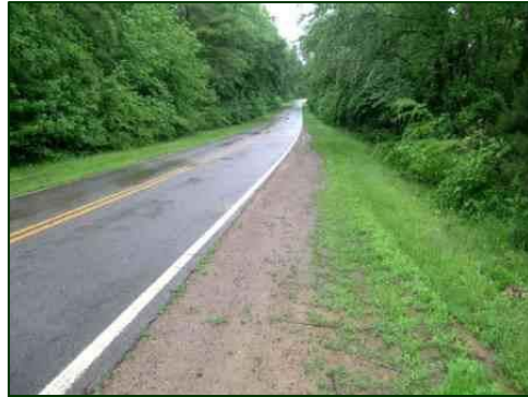
Figure 2. Look back view of the roadway.
