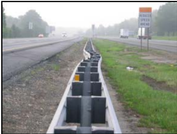
Figure 3: Eastward lookback view along the guardrail.
