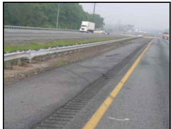
Figure 4: Westward view of the roadside departure and guardrail impact.
