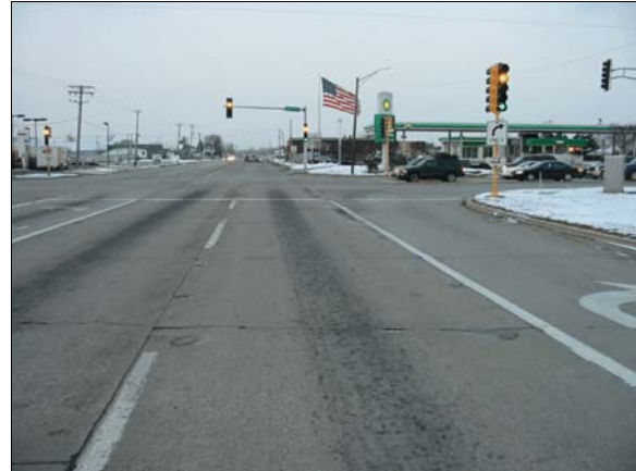
Figure 2: Approach of the Oldsmobile northbound in outside through lane
