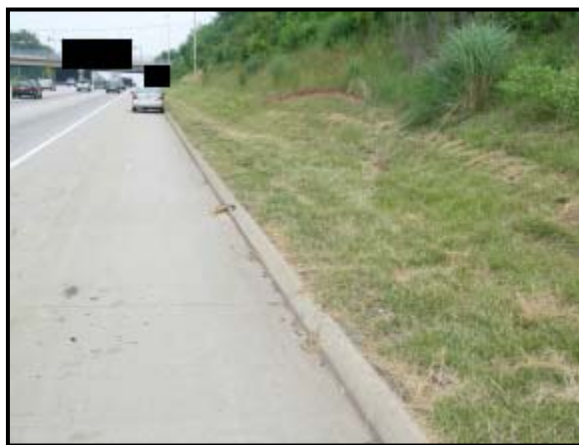
Figure 3: View at the point of roadside departure.
