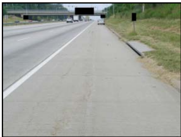
Figure 2: Eastbound view of the roadway.
