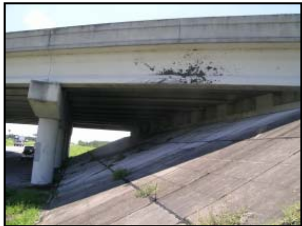
Figure 6: Overpass impact and final rest.
