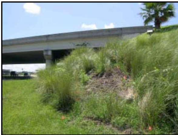
Figure 5: Southbound trajectory view at the embankment
