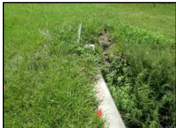
Figure 4: Concrete headwall, delineator post and gouge.
